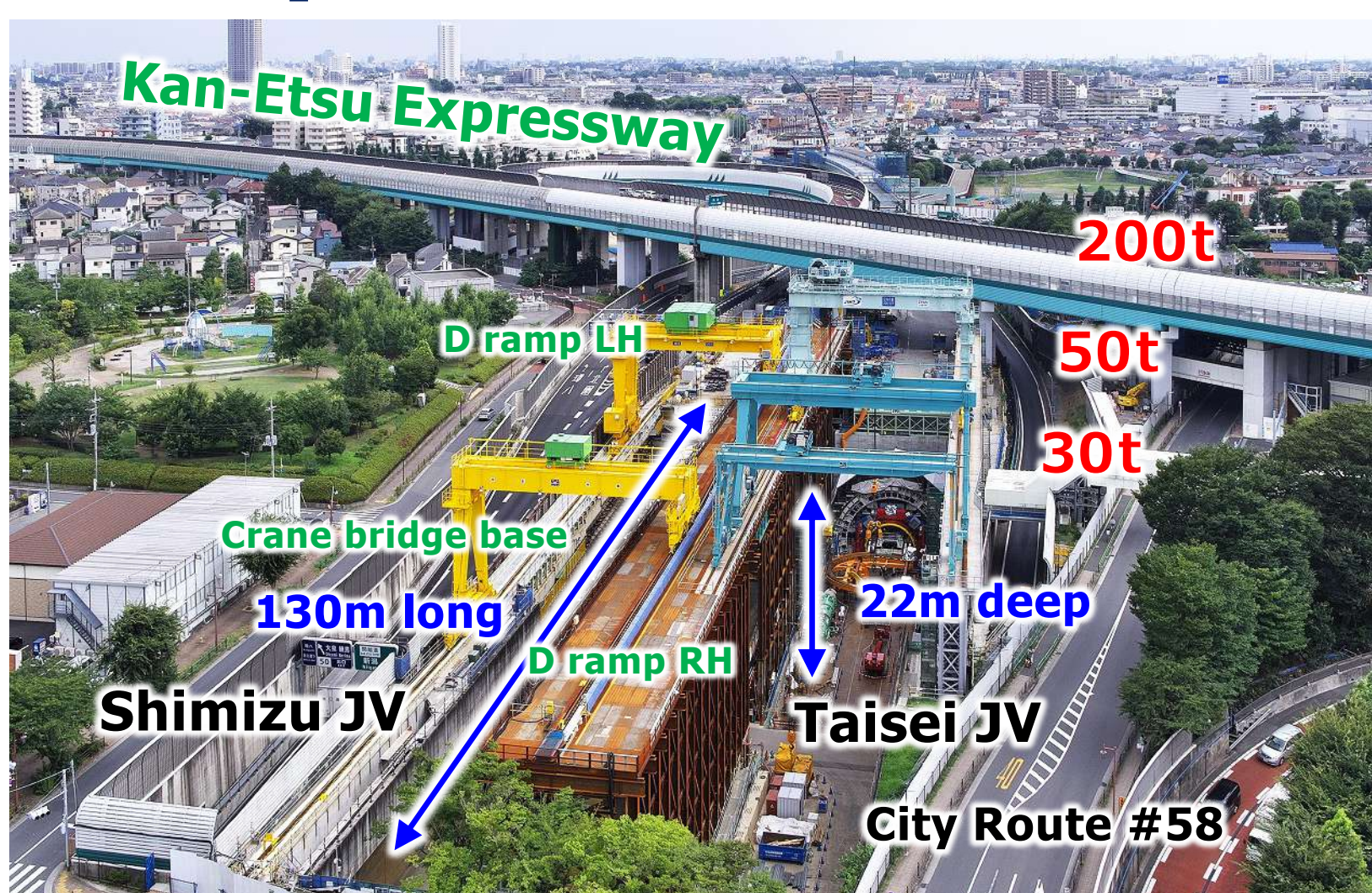
Temporary installation of the starting vertical shaft
