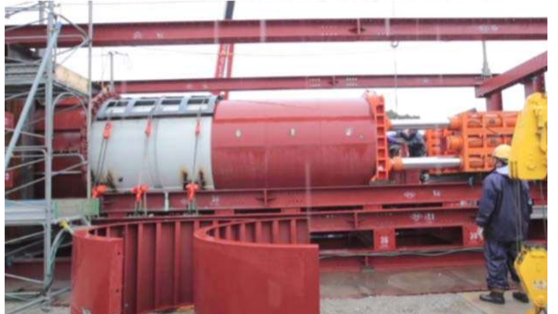
Testing (cutting through a simulated soil layer inside shaft)
