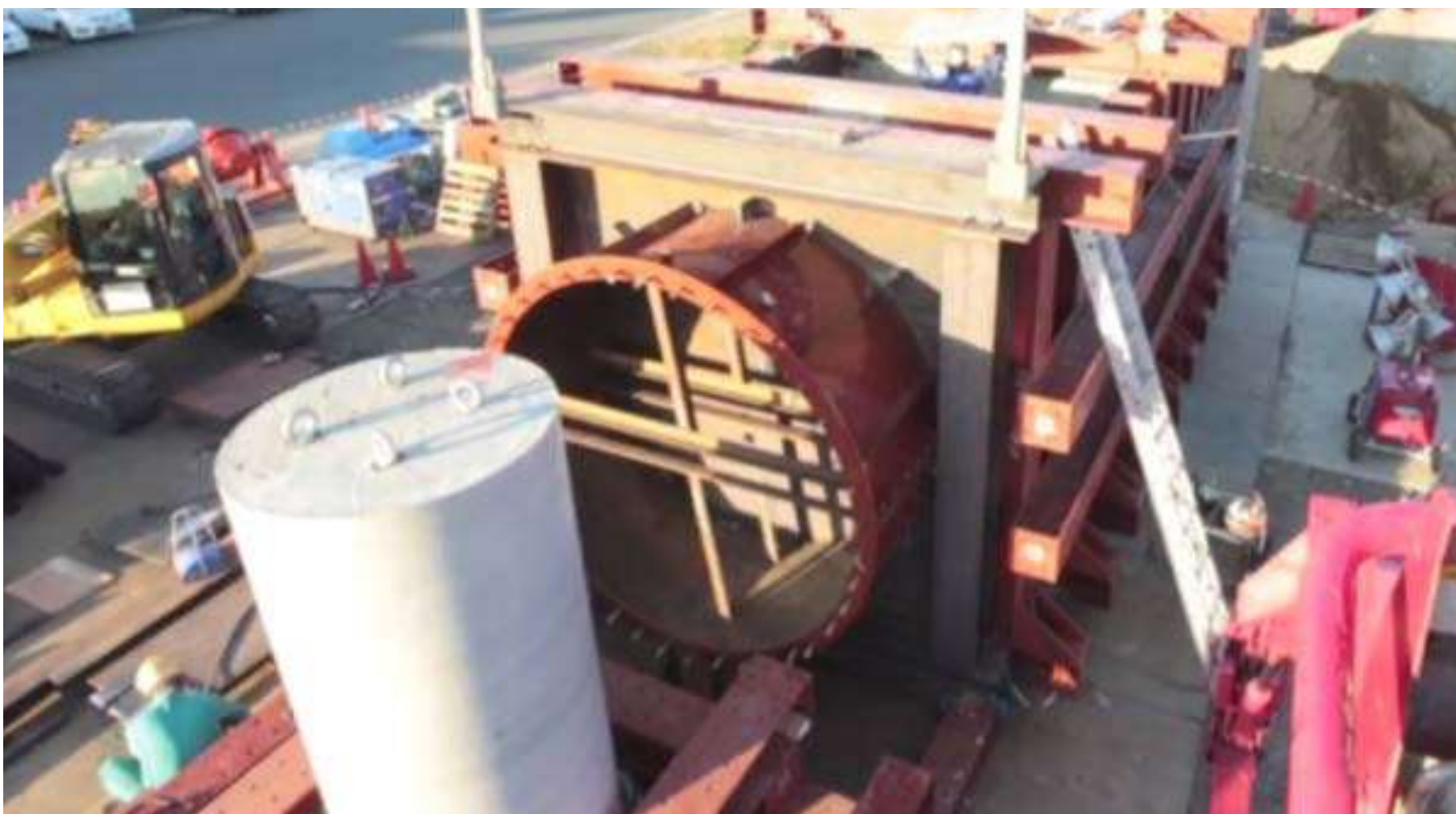
Testing (simulated single pile being cut)
