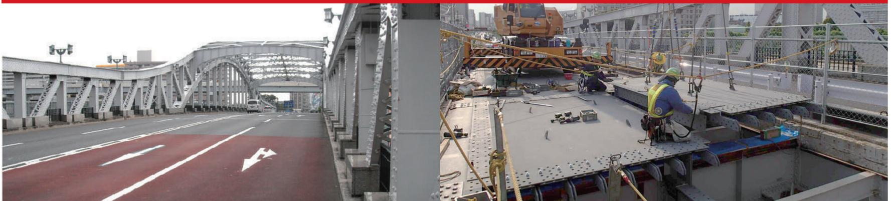
When first built in 1931 the Shirahigebashi Bridge was a reinforced concrete base structure, but was renewed in 1989 to a grating floor base construction. After further antiseismic and other reinforcement features were added in later years, the bridge was again updated from the grating floor base structure to a steel floor base structure to reduce dead weight to reduce anticipated seismic stress on the piers in the event of earthquake.
