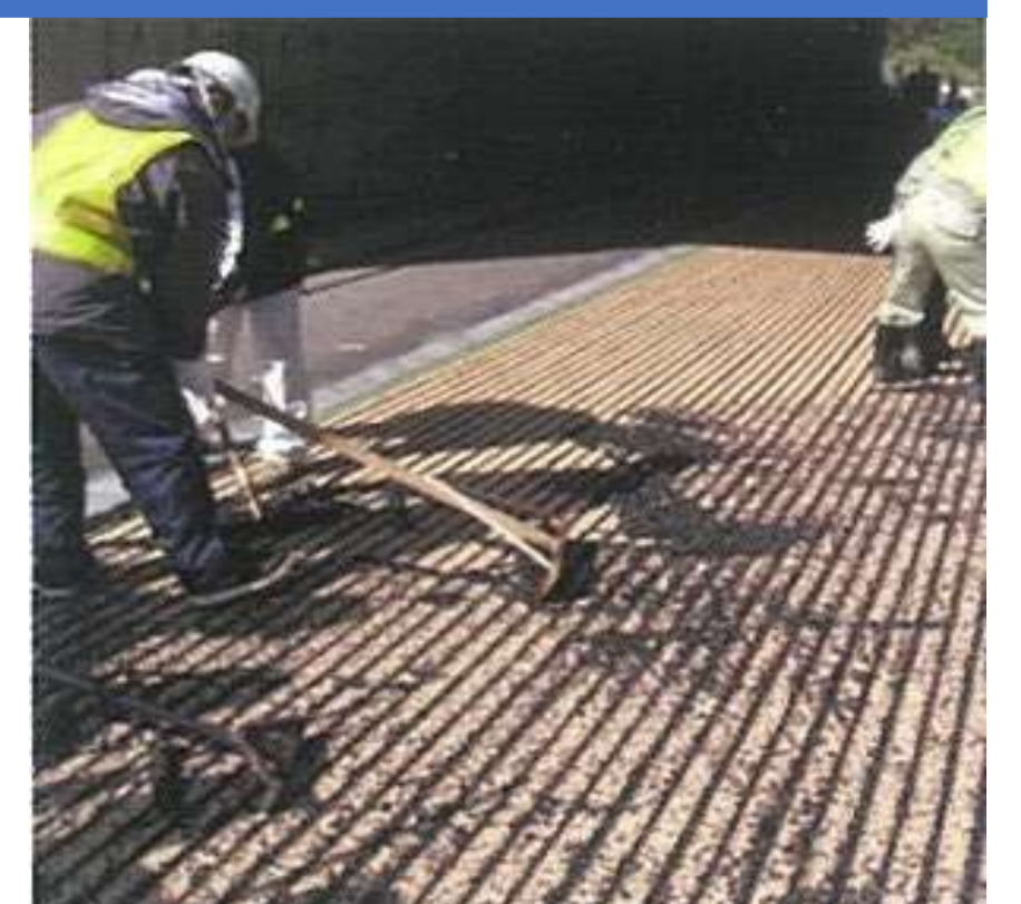
4. Injecting the freezing prevention mix
