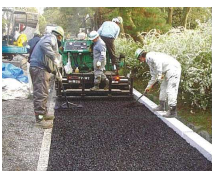
1. Laying and leveling special asphalt
