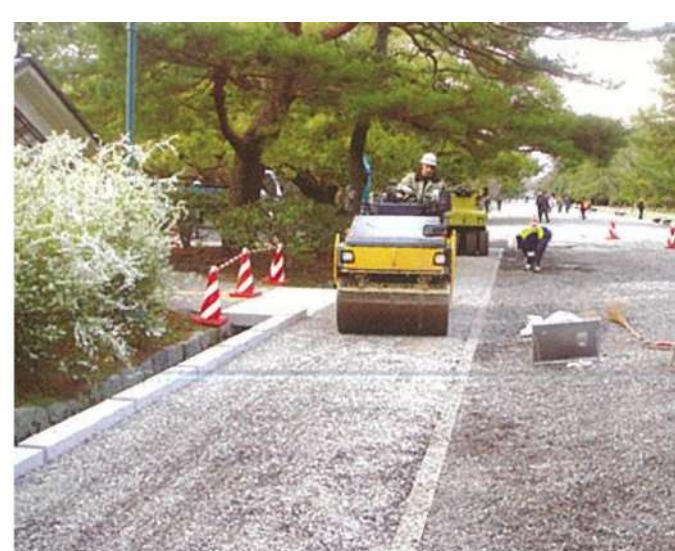
3. Compacting and rolling the pebbles
