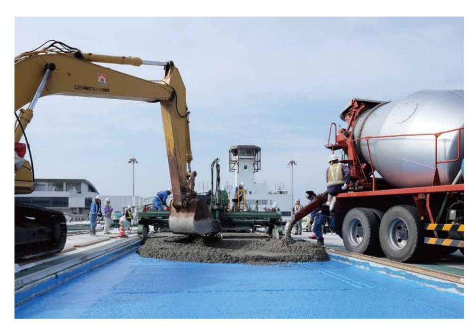
2 Concrete Overlay Construction Method with Adhesives to adjust the inclination in Airports.
