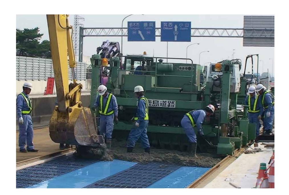
1 Concrete Overlay Construction Method with Adhesives and SFRC To Extend a life of Orthotropic Steel Deck Bridges.
