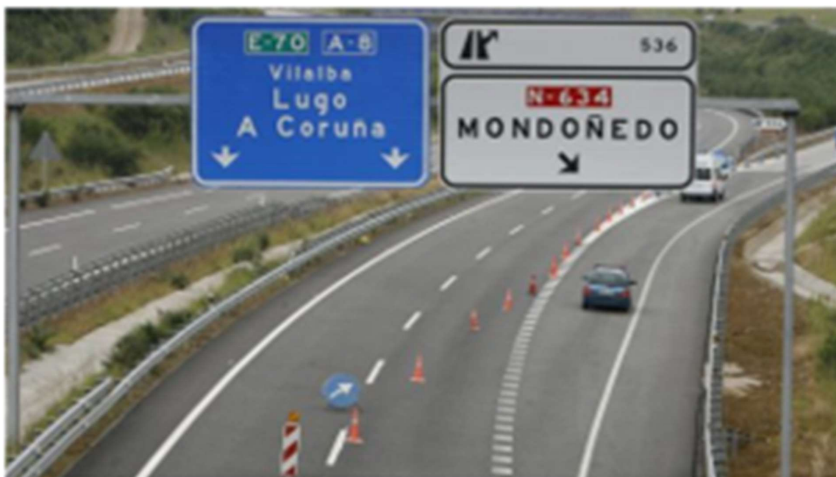
Figure 4 - Manual detour by means of physical lane markings on A-8.
