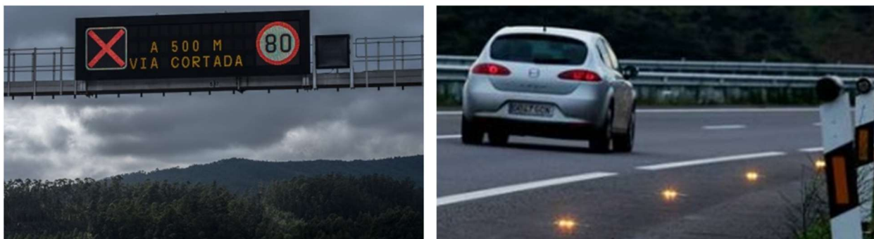
Figure 8 – Variable Message Sign and pavement markings. A-8 Motorway. Alto del Fiouco (Lugo). Spain
