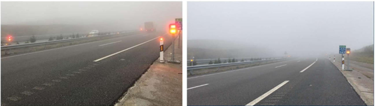
Figure 11 - Detector beacons in low visibility conditions. A-8 motorway. Alto de O Fiuoco (Lugo). Spain
