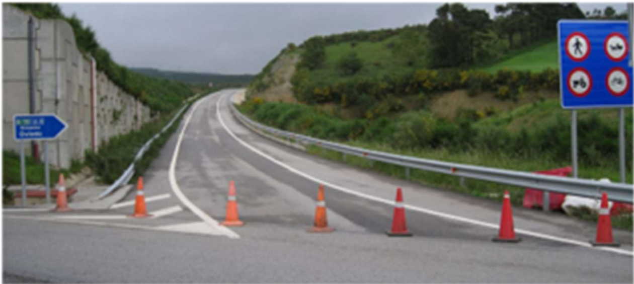
Figure 5 - Manual detour by means of physical signalling on access to A-8
