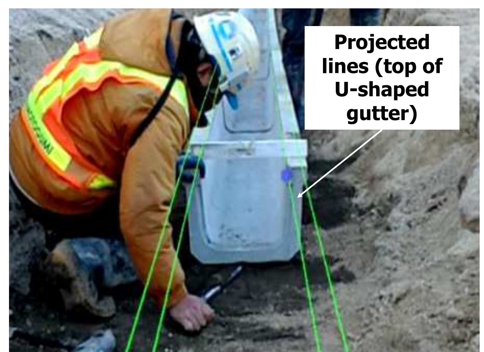
AR image overlay with a wearable device
