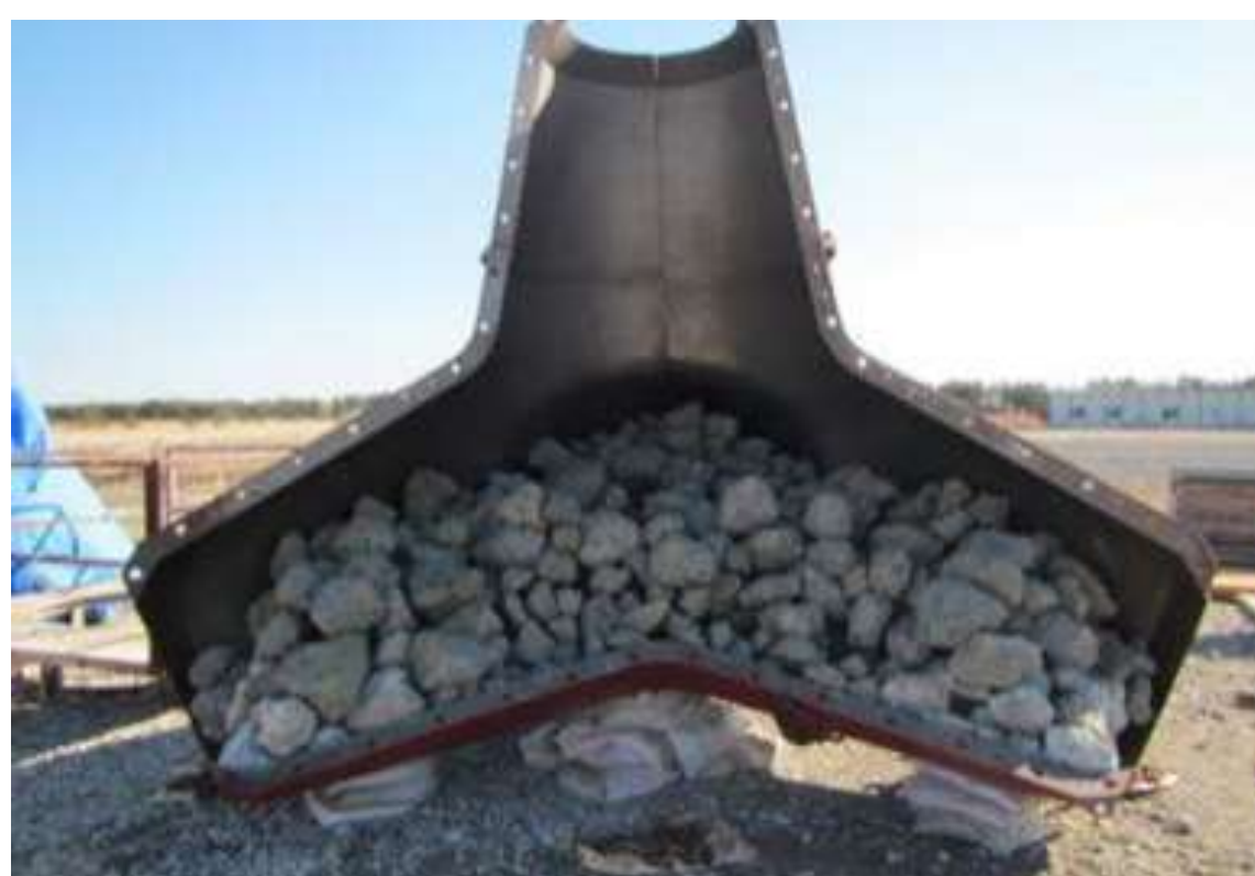
Prepacked concrete block using concrete debris
