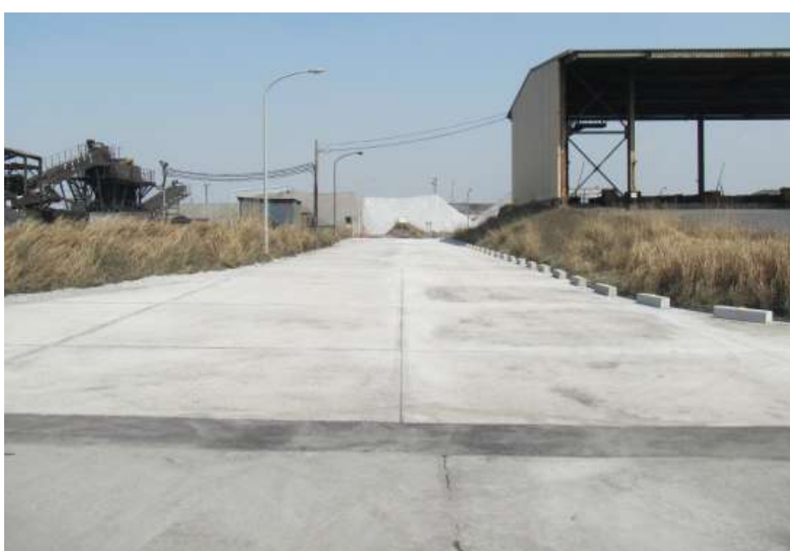
Pavement using blast furnace slags
