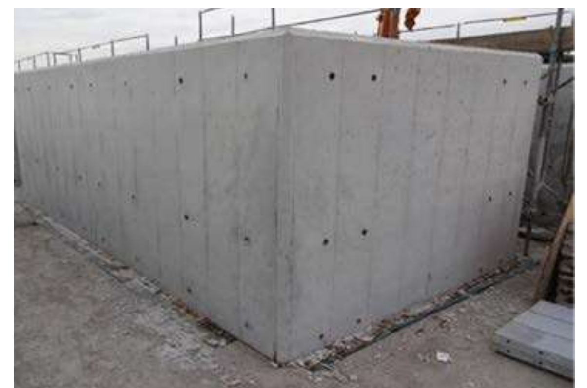
Revetment block for seaport protection
