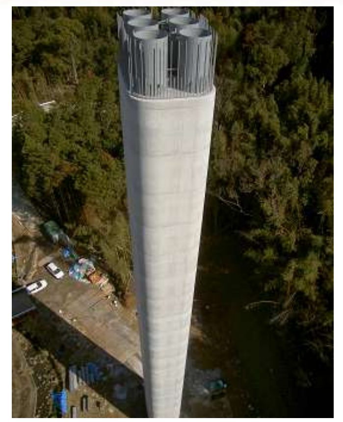
Steel-pipe-and-concrete composite bridge pier
