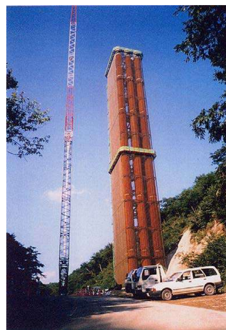
Steel pipe and reinforcement assembly completed
