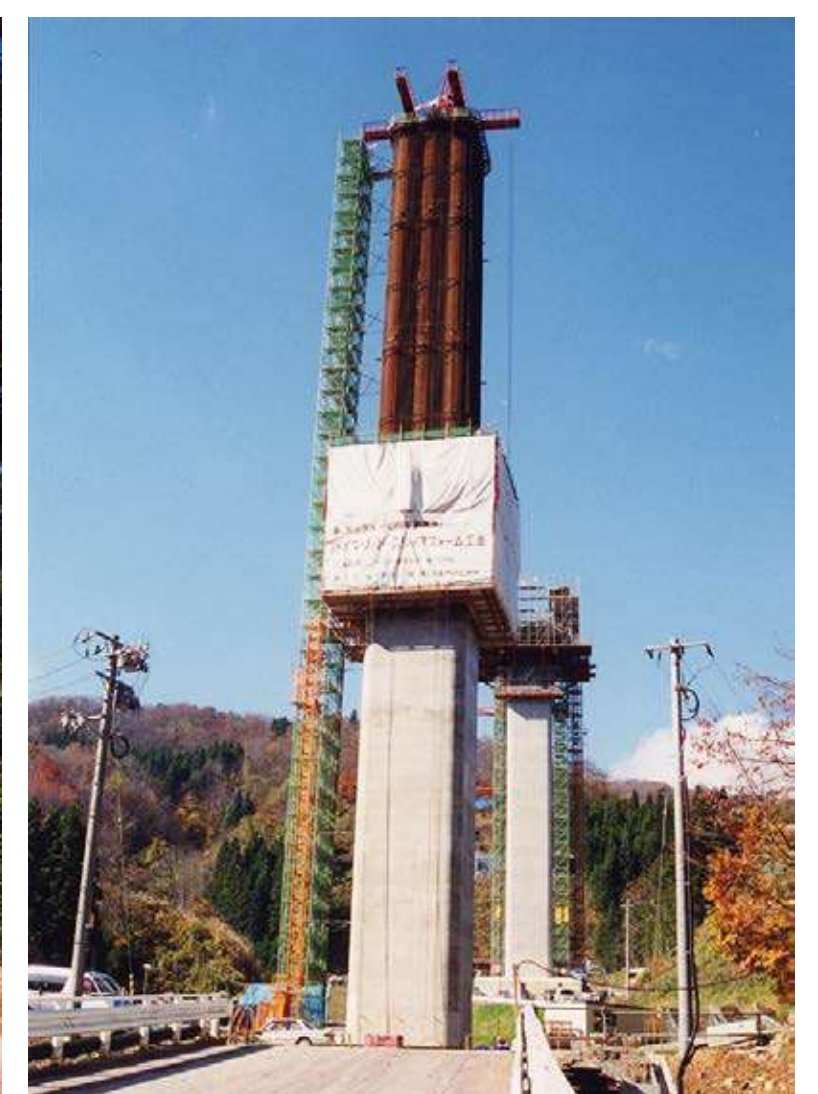
Slipform system in operation
