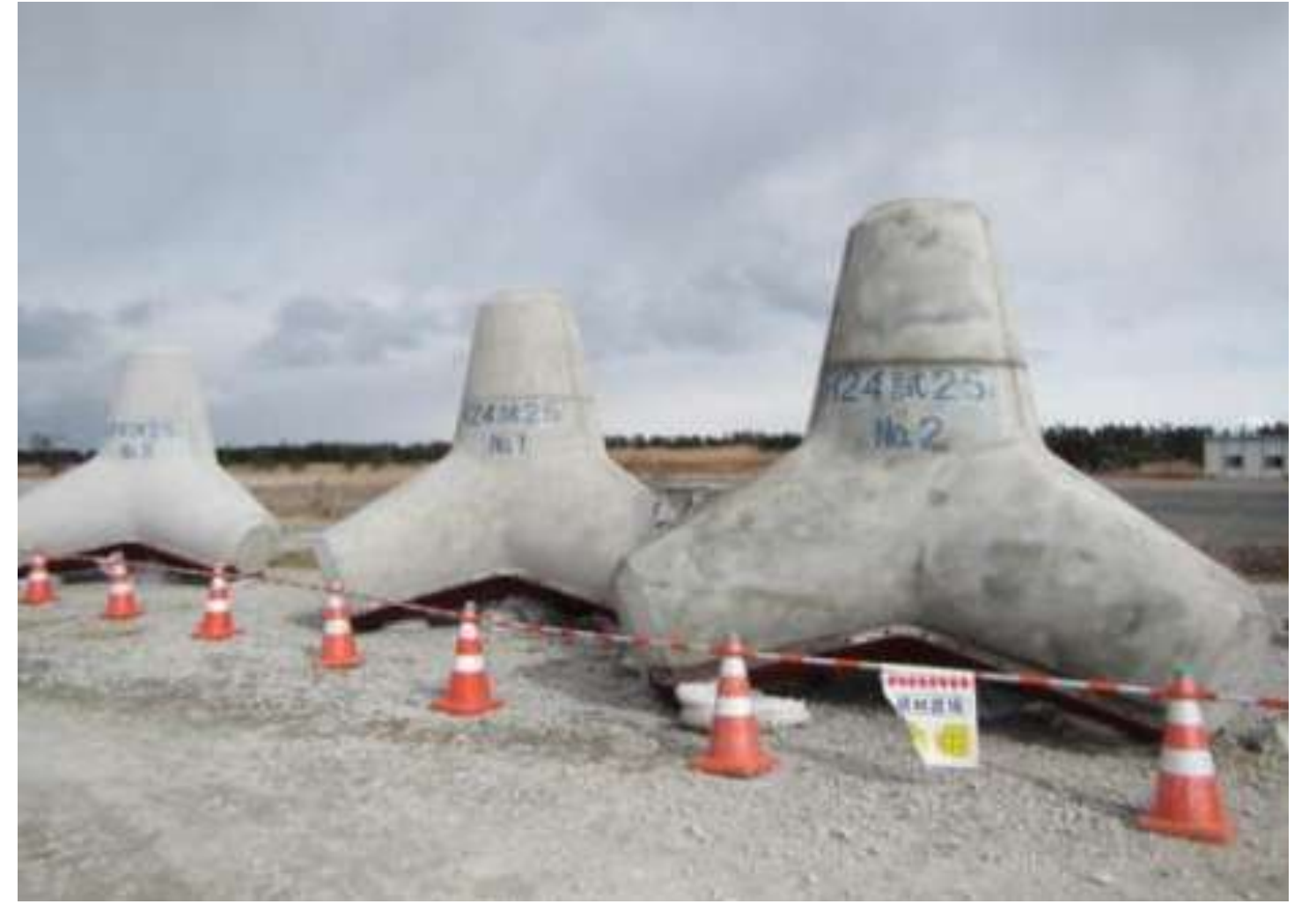
Wave-dissipating block fabrication as part of post-disaster restoration effort (Soma Port, Fukushima Prefecture)
