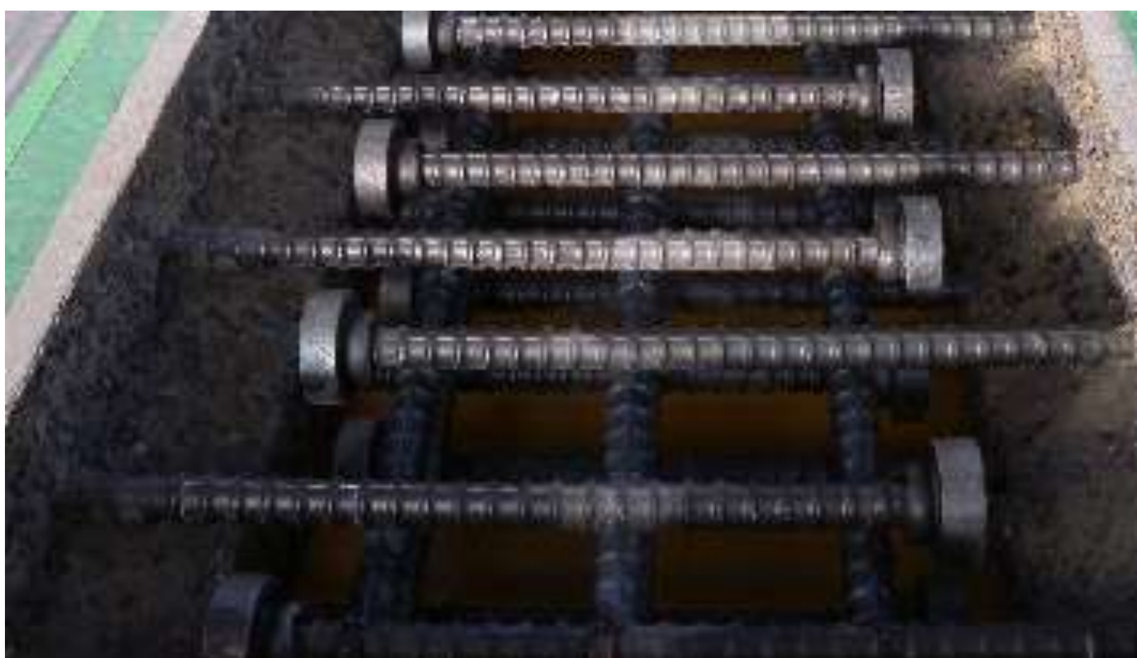
Conventional jointing method (W≈400 mm)
