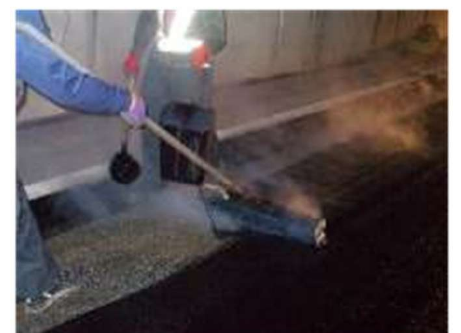
Application of membrane
