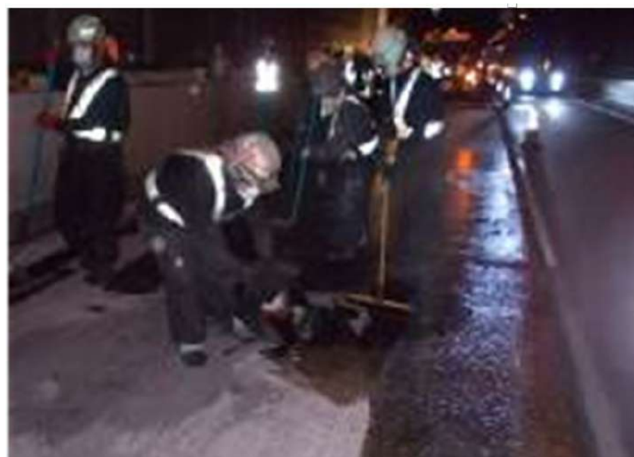
Application of Multi-Primer
