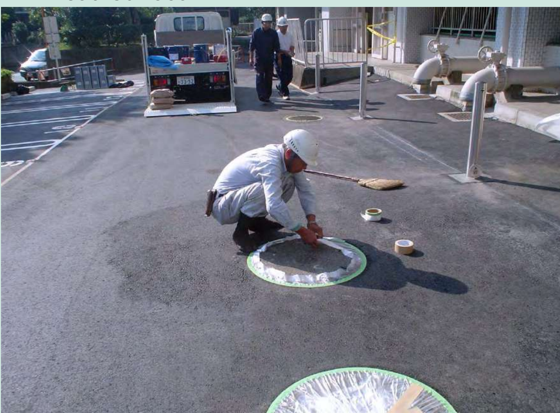
① Cleaning and Masking of existing Road Surface
