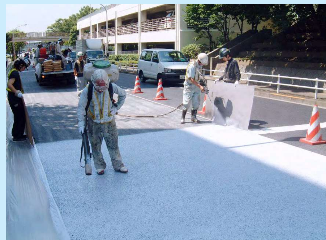
② Spraying Slip-resistance Aggregate
