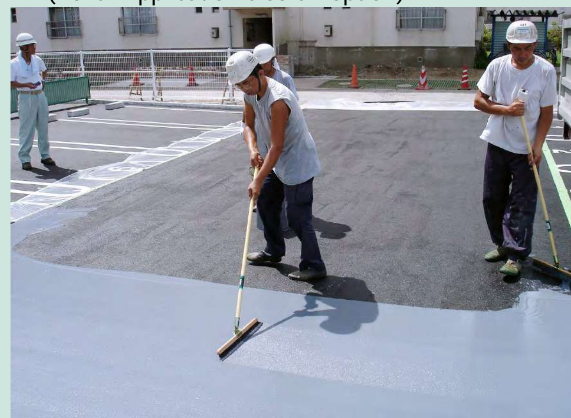
② Coating 1st Coat using Universal Broom (Roller Application also an option)
