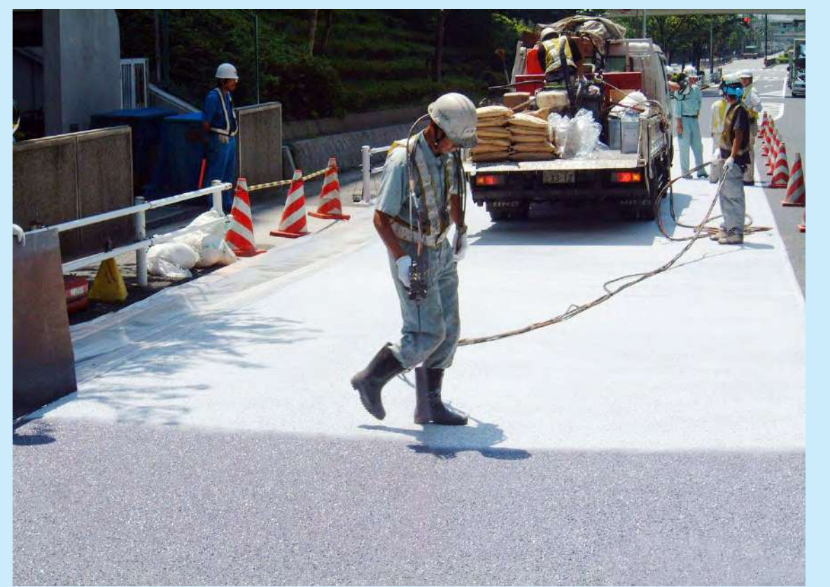
③ Spraying 2nd Coat
