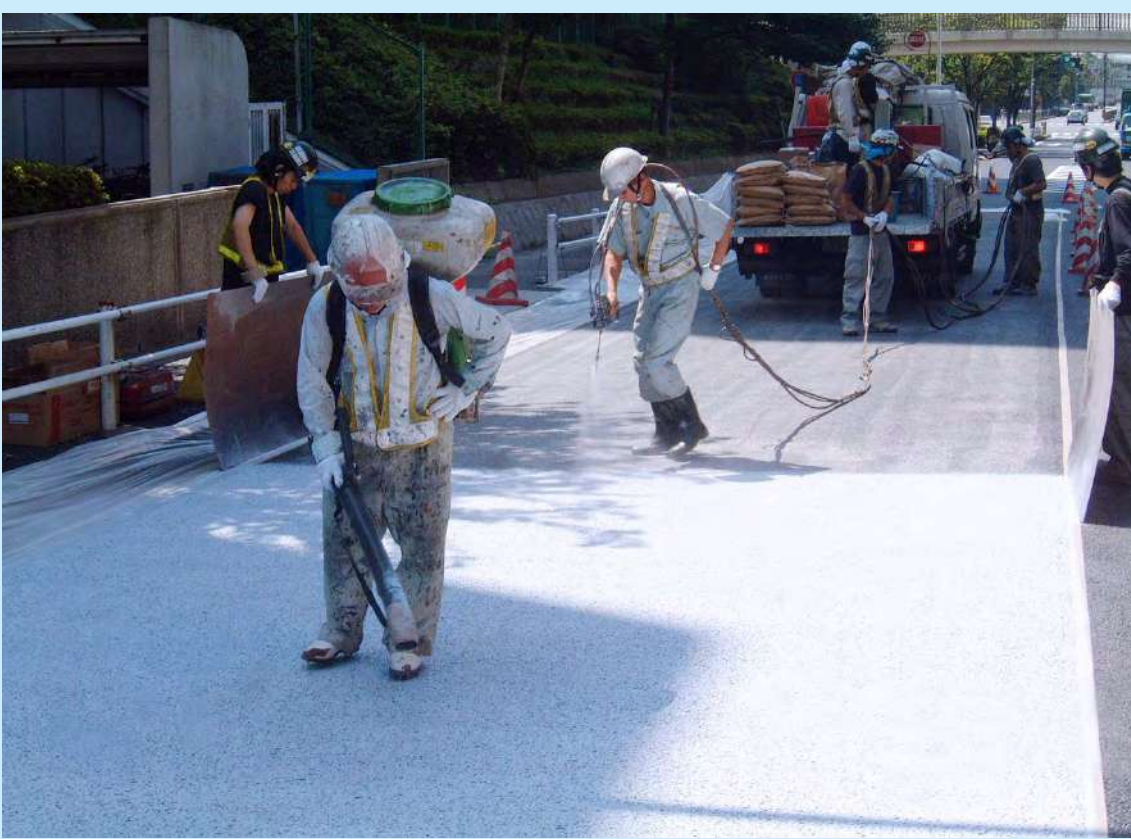
① Spraying 1st Coat with specialized Sprayer
