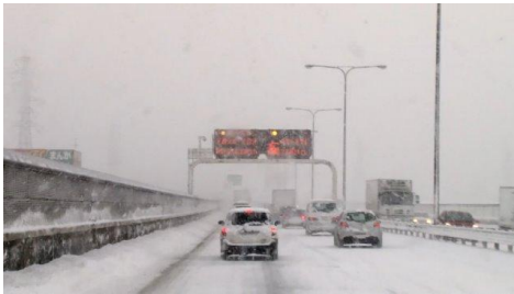
Expressway road surface condition in winter
