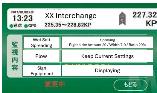
Integrated control panel screen
