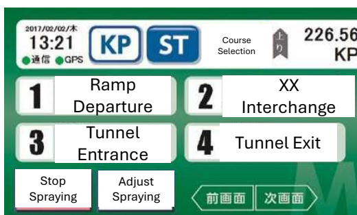
Integrated control panel screen
