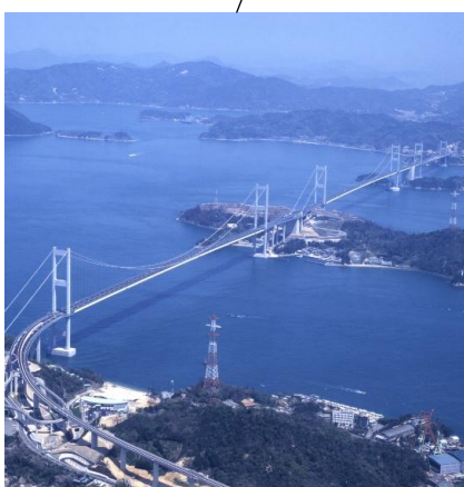
Kurushima Kaikyo Bridges (Open 1999, Length 4,106 m)
