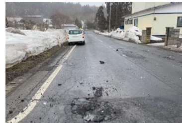
Early detection of potholes during the snowmelt season
