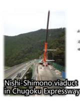
Replacement of precast concrete decks
