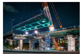
Single-operation erection of superstructures (Chugoku Expressway Renewal)
