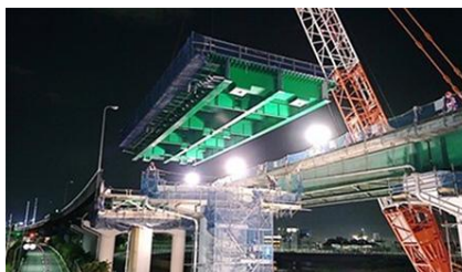
Erection by a Crane
