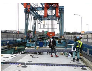
Deck Replacement by a Gantry Crane (at Low Clearance)
