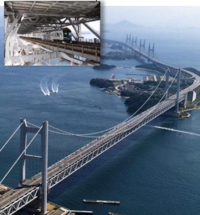
Seto-Ohashi Bridges (Open 1988, Length 9,360 m)
