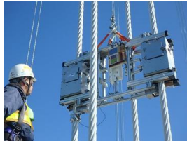
Suspender rope inspection
