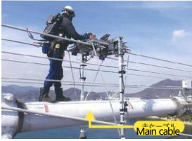
Main cable inspection
