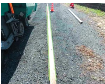
AI system tracking the formwork
