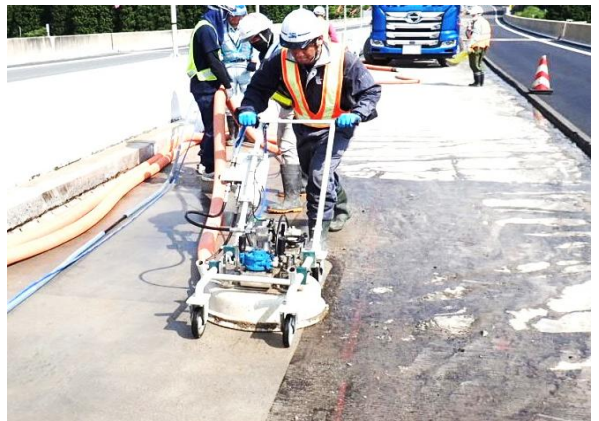
Deck slab cleaning (small unit)
