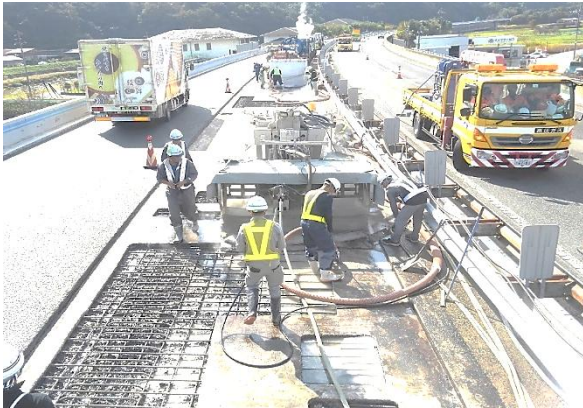
Hydro-milling operation (front view)
