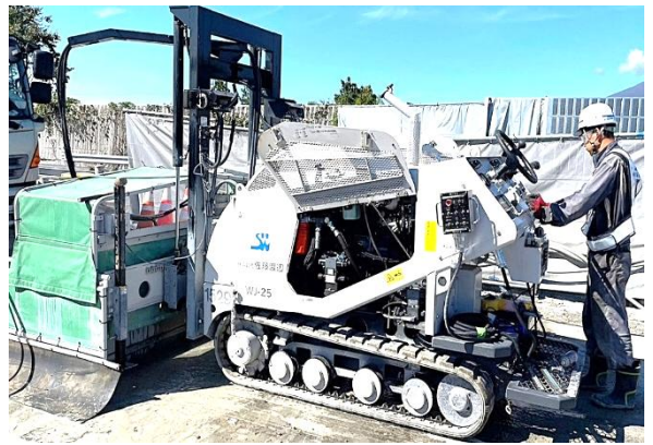
Hydro-milling operation (side view)
