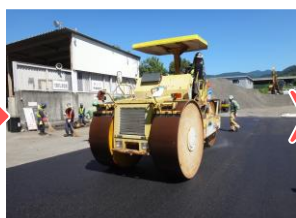
Initial compaction
