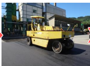
Final compaction
