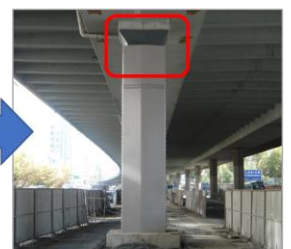
Lead rubber bearing installed. Work completed
