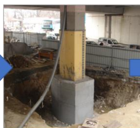
Concrete lining installed on the underground part
