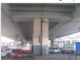
Steel lining plate installed around the existing PC pier
