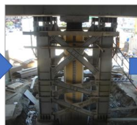
Pier head cut while supported by a steel bent
