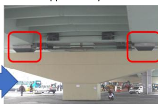
Pier head cut while supported by a steel bent
