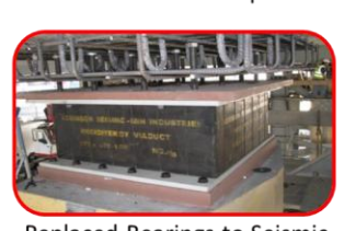
Replaced Bearings to Seismic lead rubber bearing
