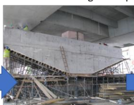
Concrete lining installed on the underground part
