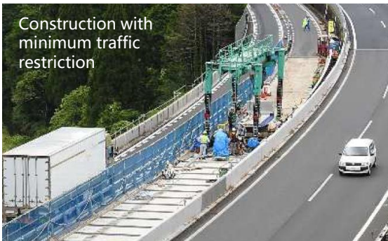
Half-slab replacement with one lane in service
