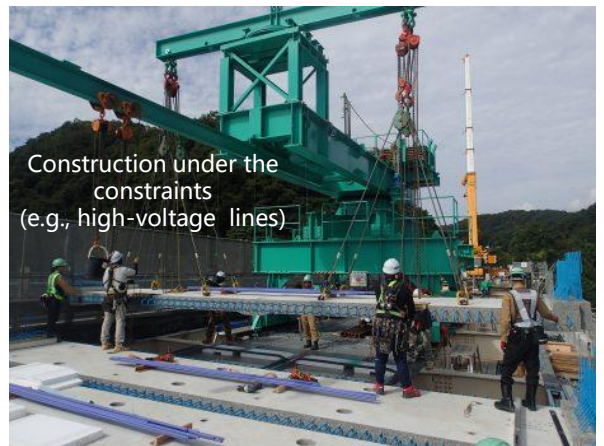
Deck slab replacement using deck slab erection equipment
