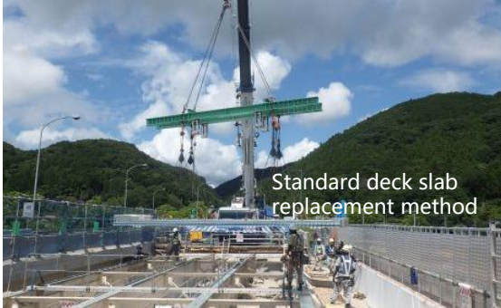
Deck slab replacement using mobile cranes
