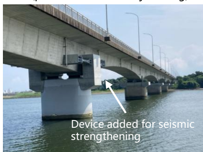
Adding seismic strengthening devices to an existing prestressed concrete bridge
