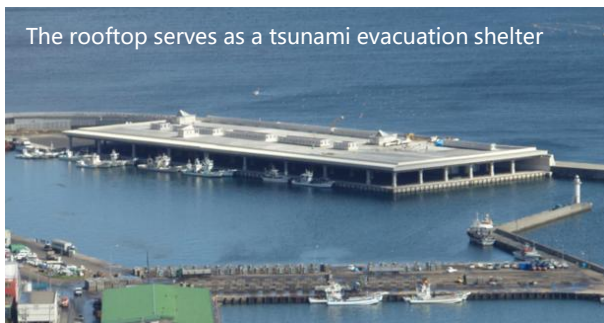
Artificial ground constructed offshore
