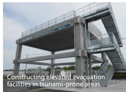
Tsunami evacuation towers utilizing PCaPC technology
