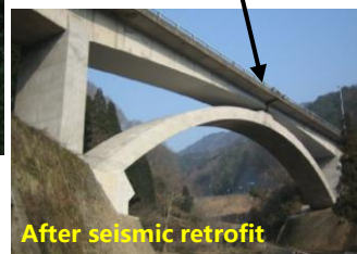
Modifying a hinged rigid-frame bridge into a continuous structure and constructing an additional arch
