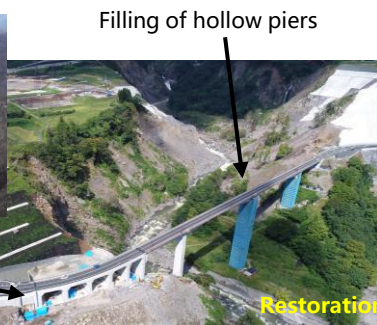
Restoration of a bridge damaged by a major earthquake
