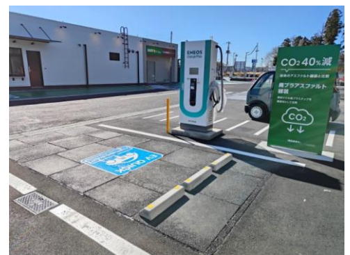
Demonstration at the ENEOS Platform Hitachino-Ushiku SS
