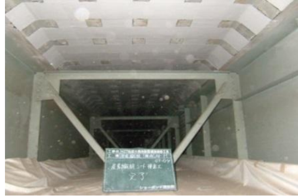
Attachment of carbon fiber sheets
