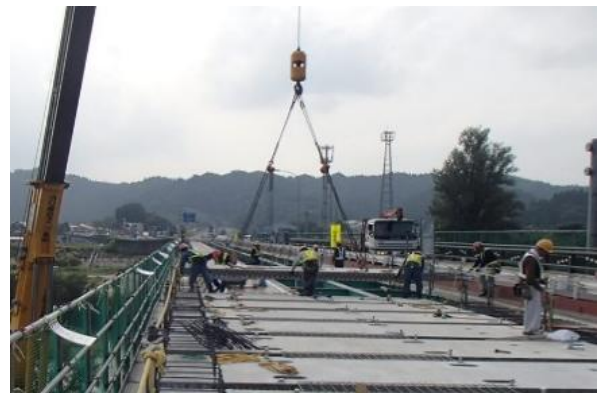
Replacement with precast deck slab
