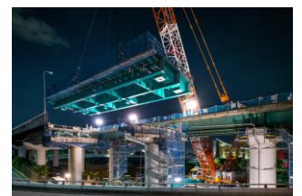
Single-operation erection of superstructures (Chugoku Expressway Renewal)
