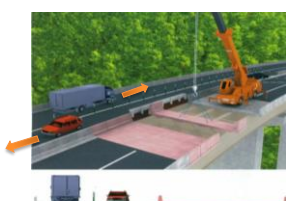
Replacement of precast concrete decks
