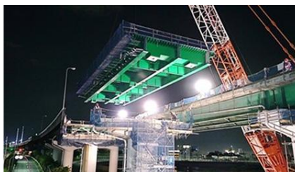
Erection by a Crane
