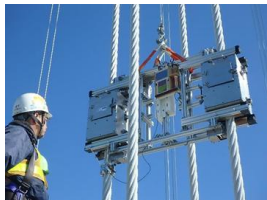
Suspender rope inspection
