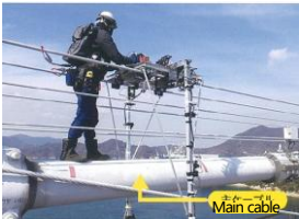
Main cable inspection
