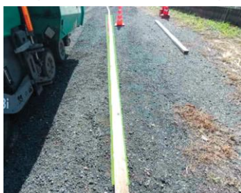
AI system tracking the formwork
