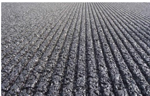
Example of longitudinally grooved rough-surface finish
