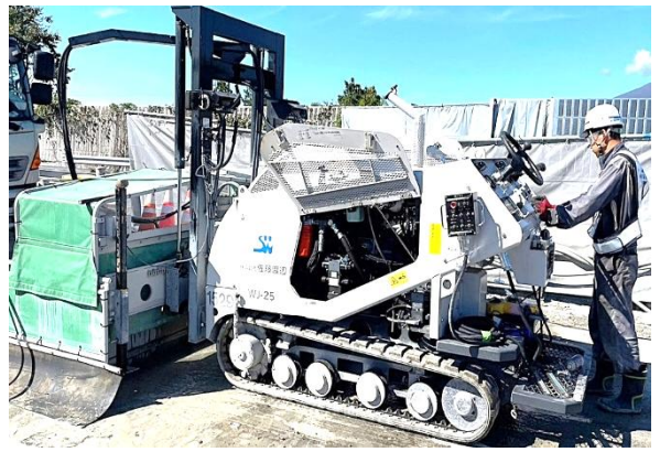
Hydro-milling operation (side view)
