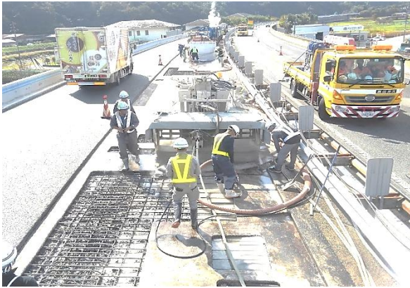
Hydro-milling operation (front view)
