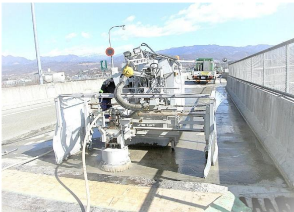
Deck slab cleaning (large unit)
