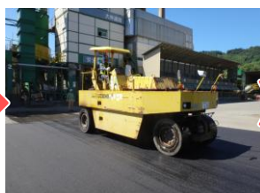
Final compaction
