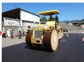
Initial compaction
