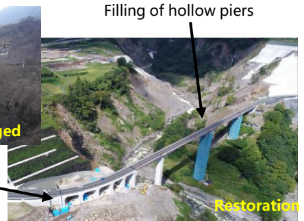
Restoration of a bridge damaged by a major earthquake
