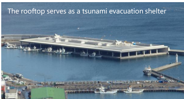
Artificial ground constructed offshore
