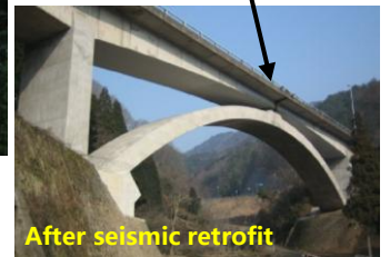
Modifying a hinged rigid-frame bridge into a continuous structure and constructing an additional arch
