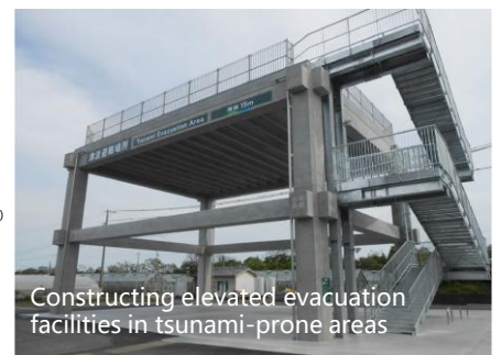
Tsunami evacuation towers utilizing PCaPC technology
