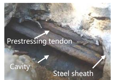
Prestressing tendon at insufficient grouting location
