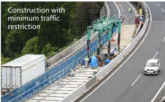
Half-slab replacement with one lane in service
