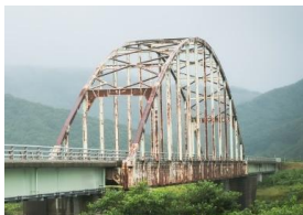
ARCH (Corrosion)
