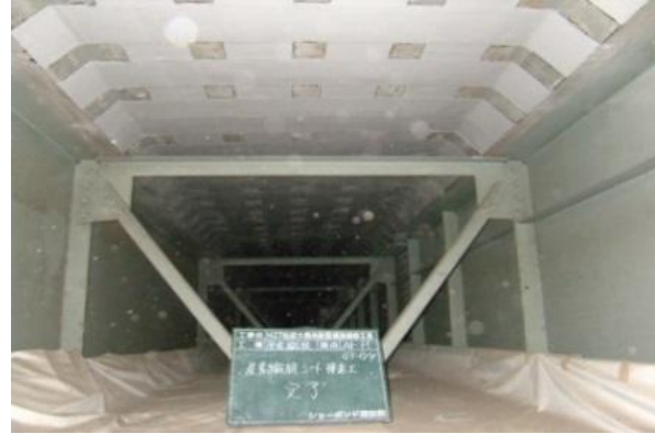
Attachment of carbon fiber sheets
