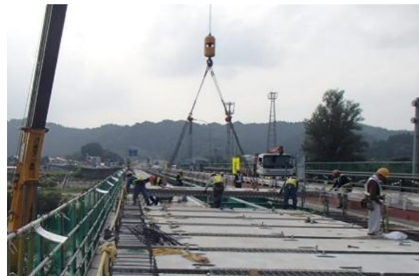
Replacement with precast deck slab
