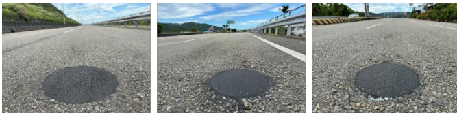
Figure 5: Example of asphalt brick application
