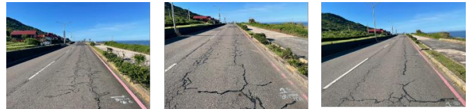
Figure 2: Example of crack sealing
