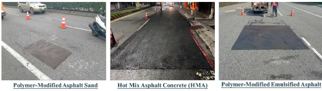
Figure 4: Example of surface sealing
