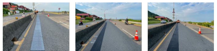
Figure 3: Example of asphalt membrane application
