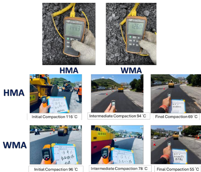
Figure 8: Field paving temperatures of HMA and WMA
