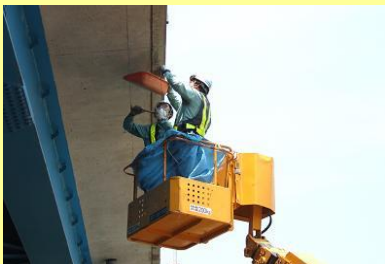
Hammering inspection for bridge
