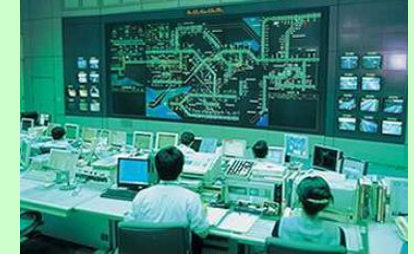
Traffic control center
