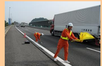
Emergency pothole repair
